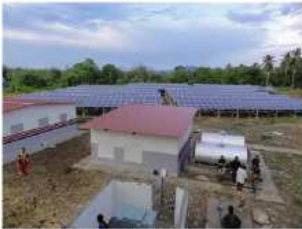
Source: IBC Solar AG, project Malaysia, 2012
